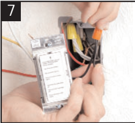
Step 7: Connect the master's Black LINE wire to the identified Line wire, usually Black, out of the wall.
